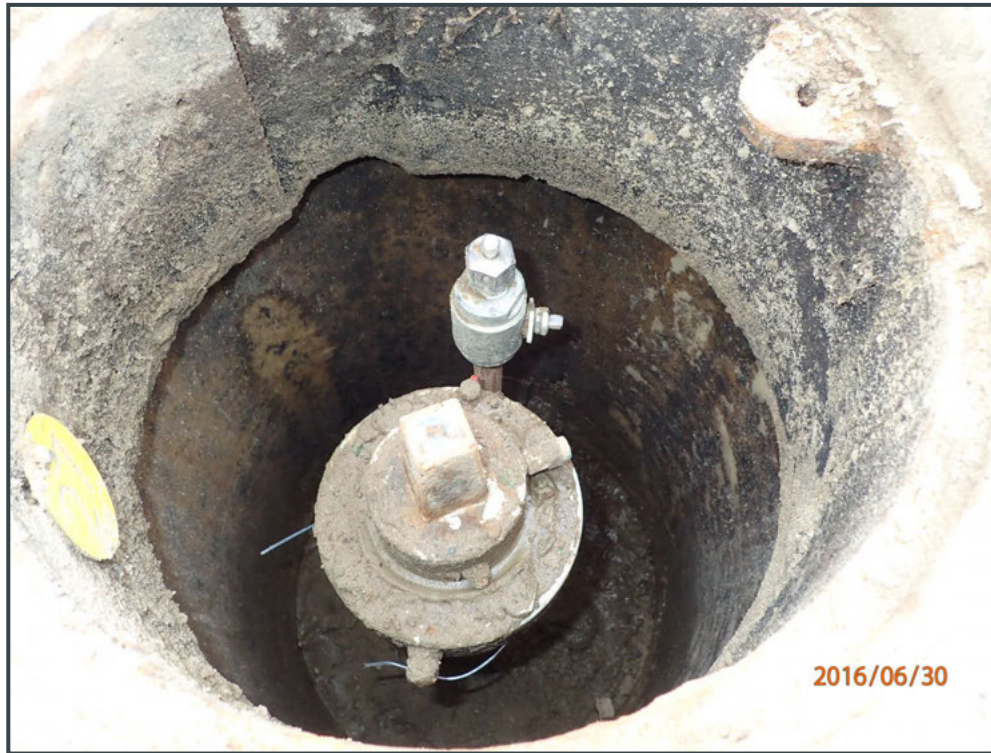
Figure 2: Example of an below ground valve of a valve location in Gasunie's medium pressure network
