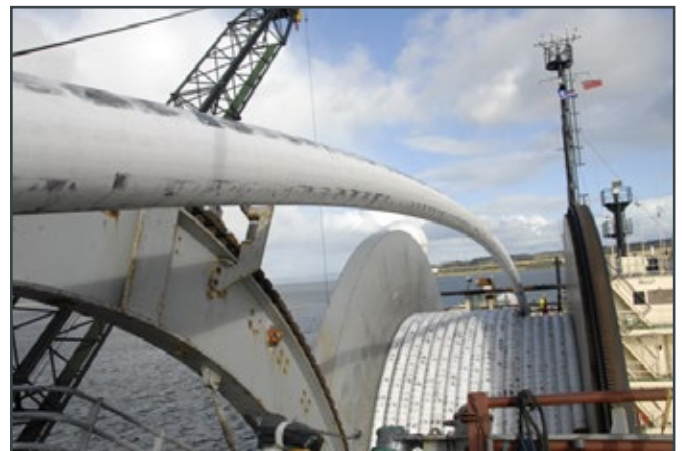
Figure 7: HFW reel lay installation onto seabed (courtesy of Tata Steel Europe)
