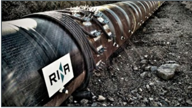
Figure 6: Test line fully instrumented
