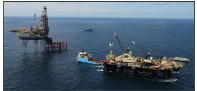
Figure 6: HFW S-lay installation onto seabed (Courtesy of Mannesmann Line Pipe GmbH)
