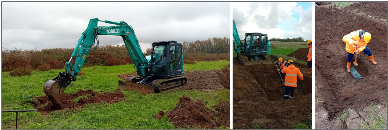
Figure 4: TPI test campaigns. Mechanical excavation (left), manual excavation (center) and impact on the pipeline shell with hammer (right).
